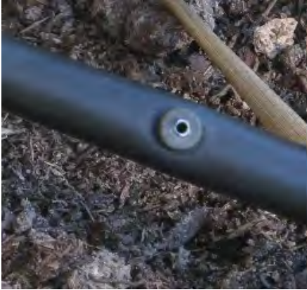
Broken transfer barb
